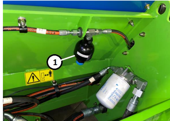
Figure 129. Accumulator Location (1) Key 1 – Accumulator
