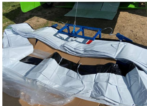
Figure 39. Bag Installation on Cradle
